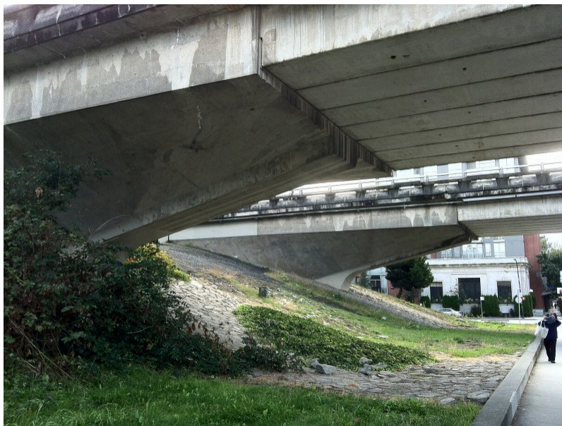
Figure 1.4 The Georgia and Dunsmuir Viaducts
