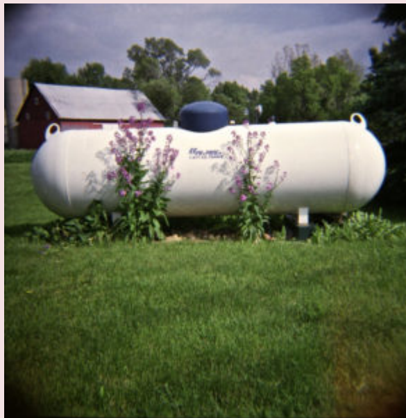
Propane is a fuel used to provide heat for some homes. Propane is stored in large tanks like that shown here.
