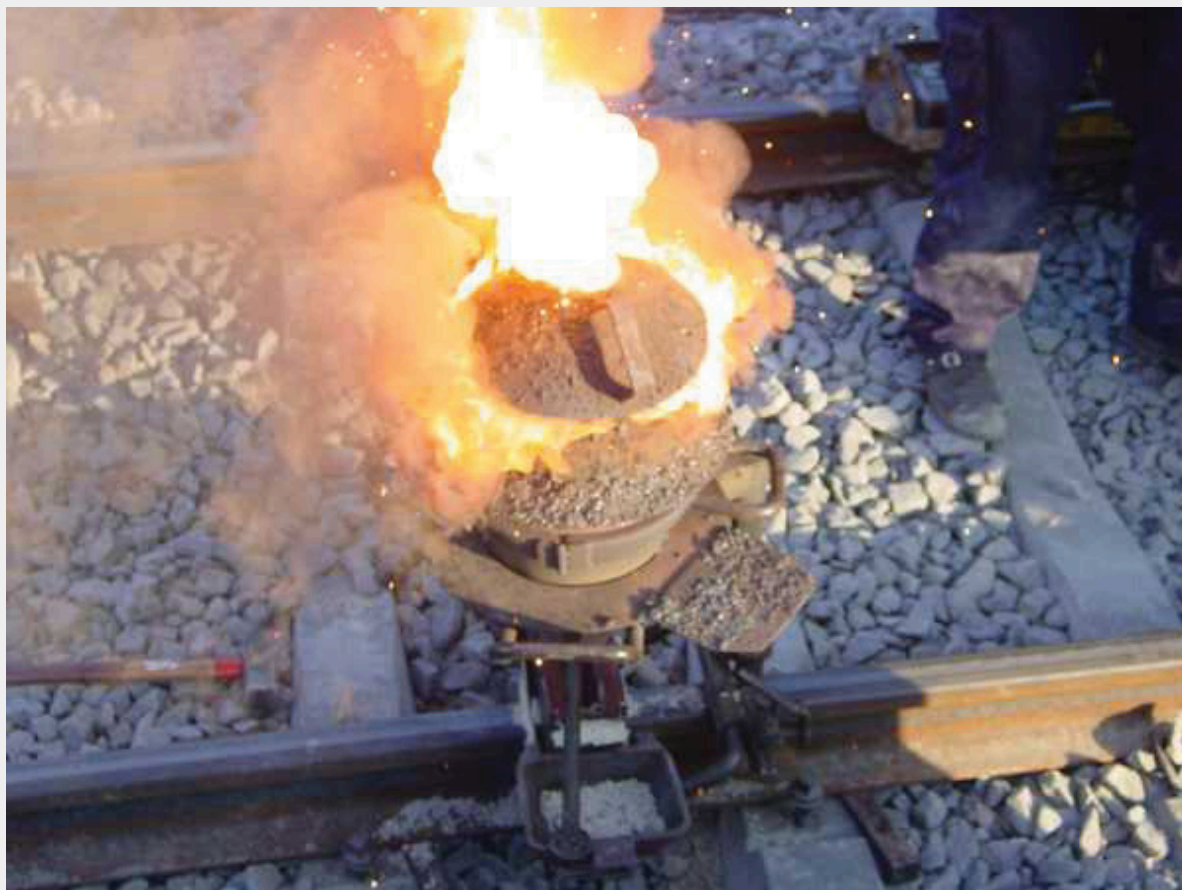
Figure 7.2 “Thermite Reaction.” A small clay pot contains a thermite mixture. It is reacting at high temperature in the photo and will eventually produce molten metal to join the railroad tracks below it.
