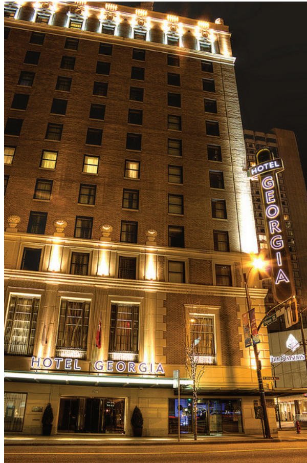
Figure 3.9 The Rosewood Hotel Georgia, a restored historic hotel in downtown Vancouver
