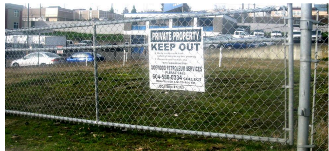
Figure 14.4.8 A closed and fenced gas station site in Nanaimo, B.C. The white pipes in the background are wells for monitoring groundwater contamination on the site.
