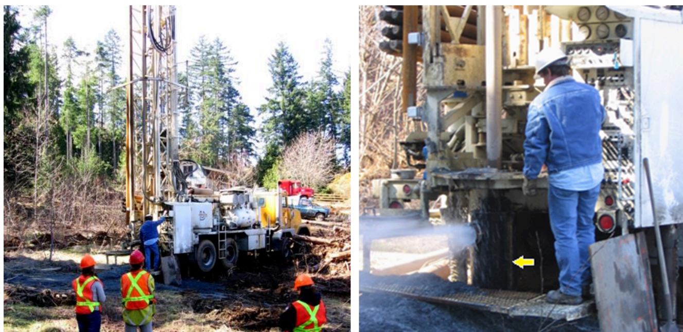
Figure 14.3.1 A water-well drilling rig in operation near Nanaimo, B.C. In the photo on the right the well is being test-pumped with air pressure. The casing (yellow arrow) is about 40 centimetres in diameter.
