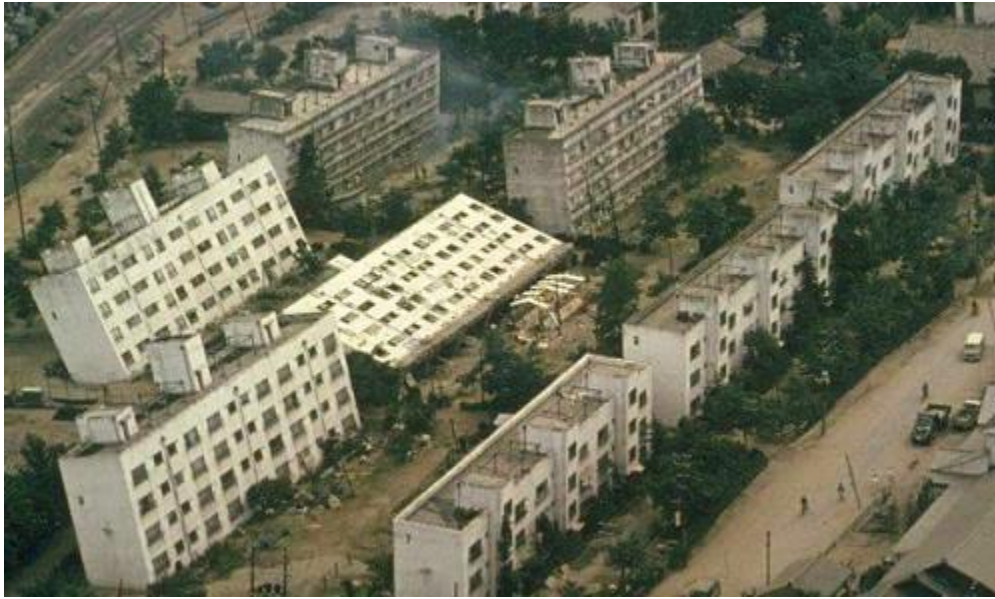
Figure 11.4.6 Collapsed apartment buildings in the Niigata area of Japan. The material beneath the buildings was liquefied to varying degrees by the 1964 earthquake.
