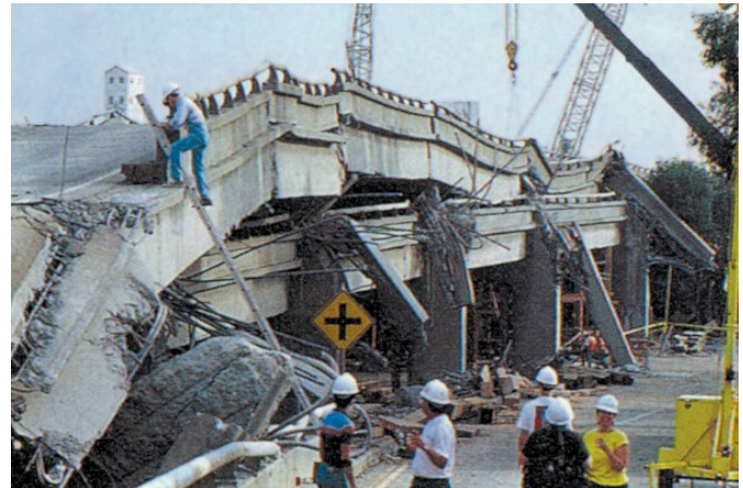
Figure 11.4.1 A part of the Cypress Freeway in Oakland California that collapsed during the 1989 Loma Prieta earthquake.
