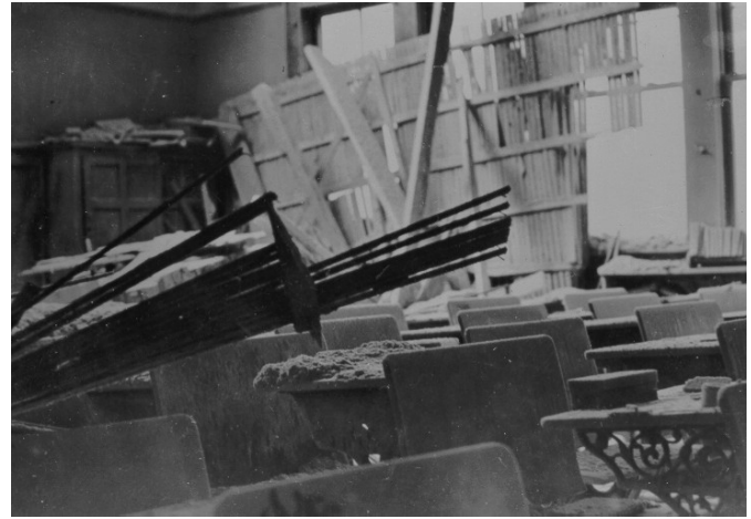
Figure 11.0.1 A schoolroom in Courtenay damaged by the 1946 Vancouver Island earthquake. If the earthquake had not happened on a Sunday, the casualties would have been much greater.
