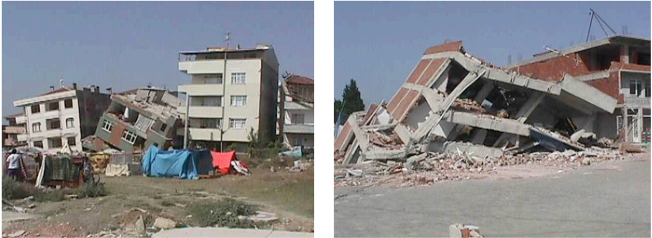
Figure 11.4.2 Buildings damaged by the 1999 earthquake in the Izmit area, Turkey.
