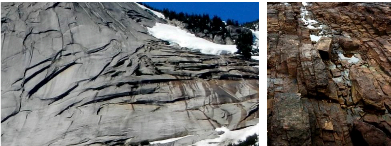
Figure 12.3.1 Granite in the Coquihalla Creek area, B.C. (left) and sandstone at Nanoose, B.C. (right), both showing fracturing that has resulted from expansion due to removal of overlying rock.
