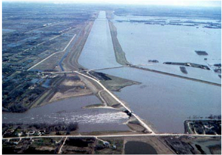
Figure 13.5.3 Map of the Red River floodway around Winnipeg, MB (left), and aerial view of the southern (inlet) end of the floodway (right).
