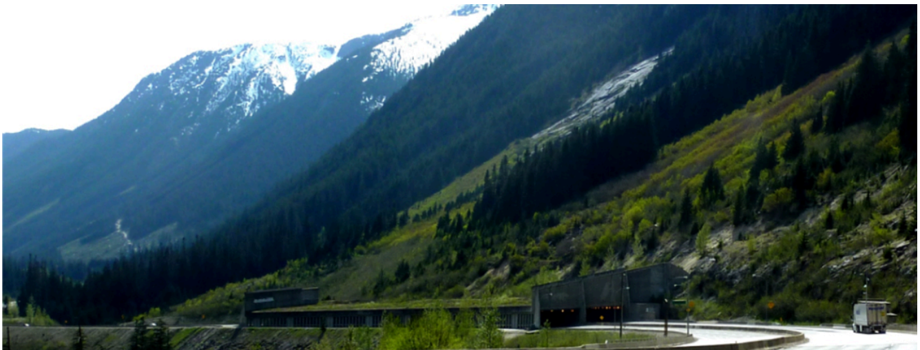
Figure 15.3.5 A snow avalanche shelter on the Coquihalla Highway. The expected path of the avalanche is the steep un-treed slope above.
