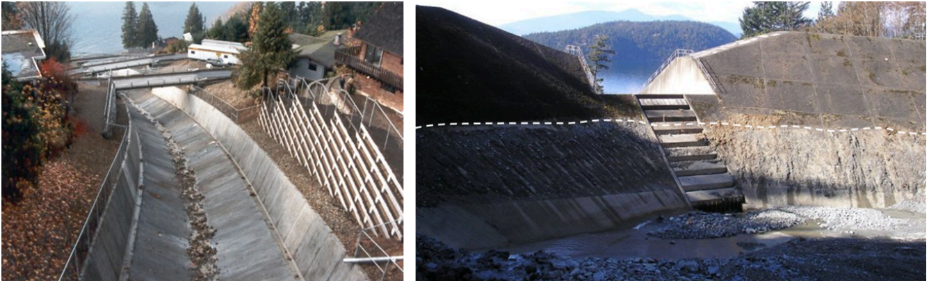
Figure 15.3.6 Two strategies for mitigating debris flows on the Sea-to-Sky Highway. Left: A concrete-lined channel on Alberta Creek allows debris to flow quickly through to the ocean. Right: A debris-flow catchment basin on Charles Creek. In 2010, a debris flow filled the basin to the level of the dotted white line.
