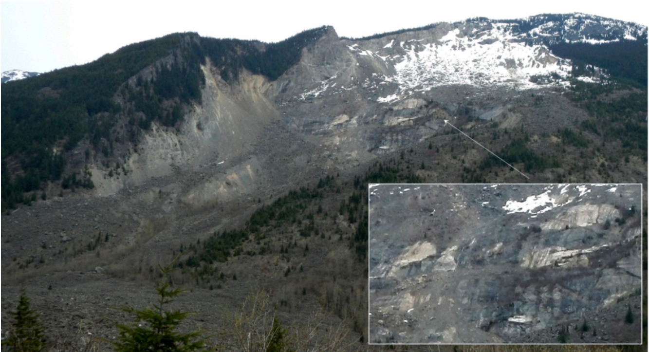
Figure 15.0.1 The site of the 1965 Hope Slide as seen in 2014. The initial failure is thought to have taken place along the foliation planes and sill within the area shown in the inset.
