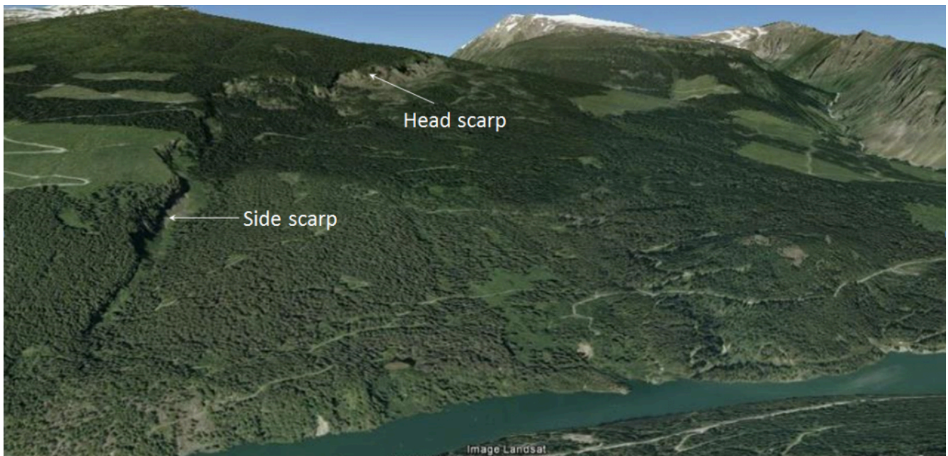
Figure 15.2.3 The Downie Slide, a sackung, on the shore of the Revelstoke Reservoir (above the Revelstoke Dam). The head scarp is visible at the top and a side-scarp along the left side.
