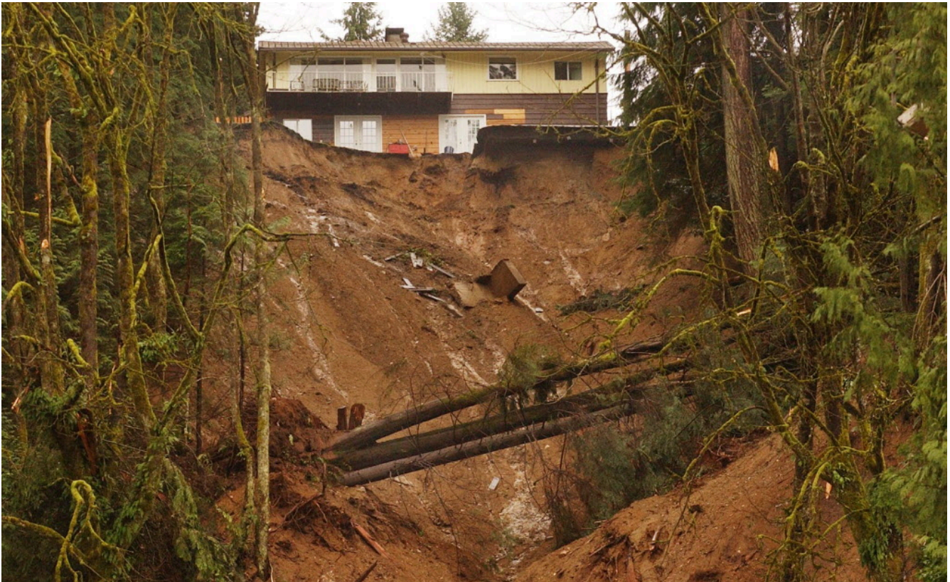
Figure 15.1.6 The debris flow in the Riverside Drive area of North Vancouver in January, 2005 happened during a rainy period, but was likely triggered by excess runoff related to the roads at the top of this slope and by landscape features, including a pool, in the area surrounding the house visible here.
