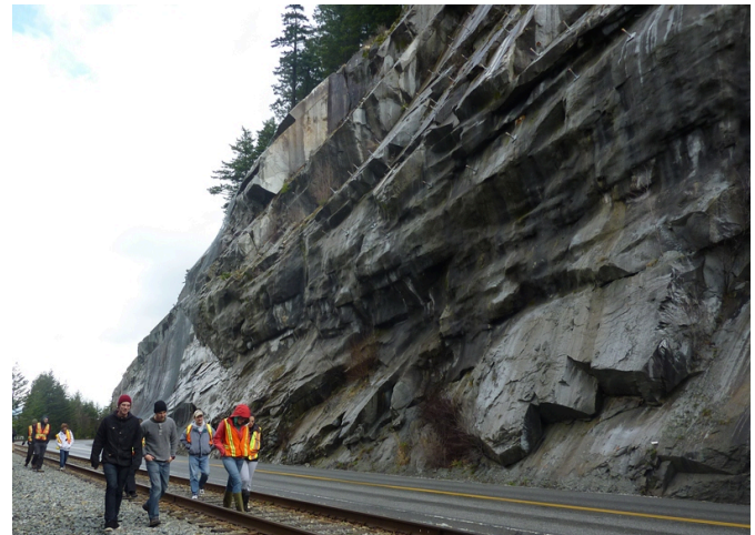
Figure 15.2.4 Site of the 2008 rock slide at Porteau Cove. Notice the prominent fracture set parallel to the surface of the slope. The slope has been stabilized with rock bolts (visible near to the top of the photo) and holes have been drilled into the rock to improve drainage (one is visible in the lower right). Risk to passing vehicles from rock fall has been reduced by hanging mesh curtains (background).
