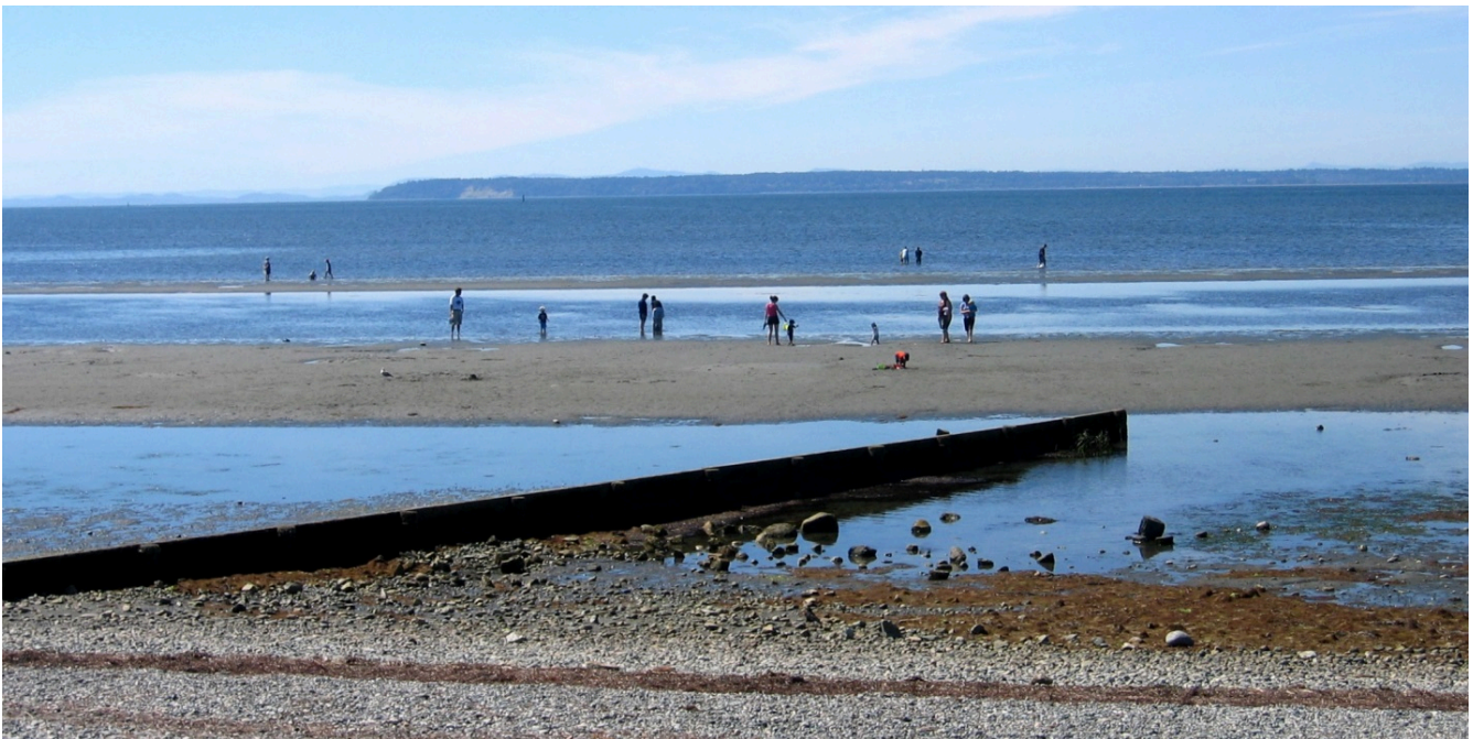
Figure 17.5.4 A groyne at Crescent Beach, Surrey, B.C.
