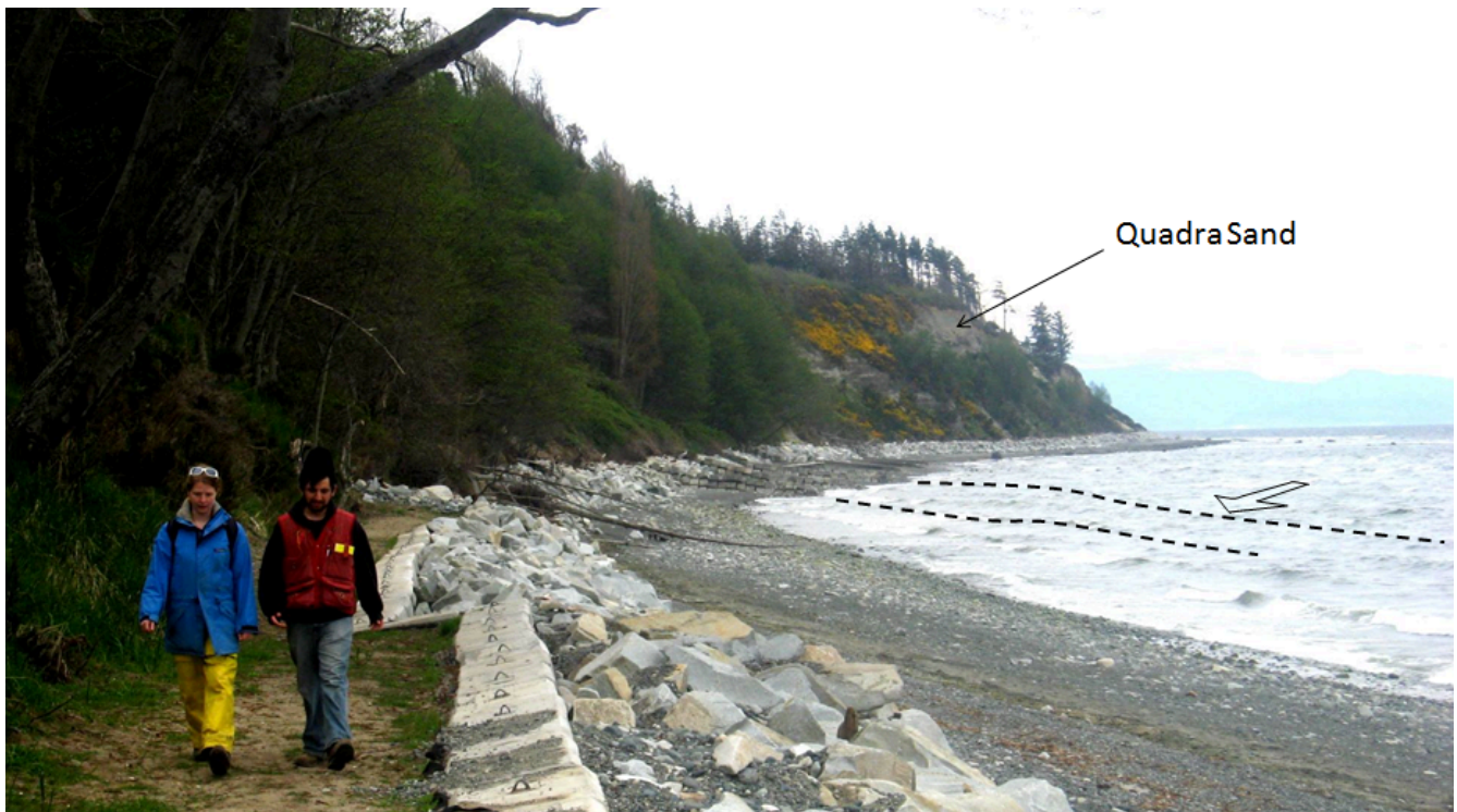
Figure 17.3.4 The Quadra Sand cliff at Comox, and the extensive concrete and rip-rap barrier that has been constructed to reduce erosion. Note that the waves (dashed lines) are approaching the shore at an angle, contributing to the longshore drift.
