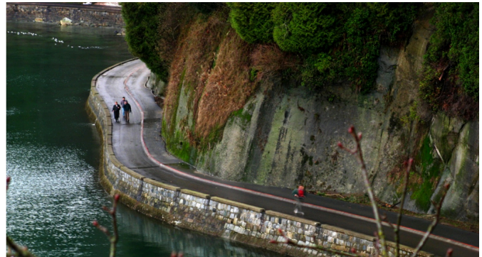
Figure 17.5.1 The seawall at Stanley Park, Vancouver.
