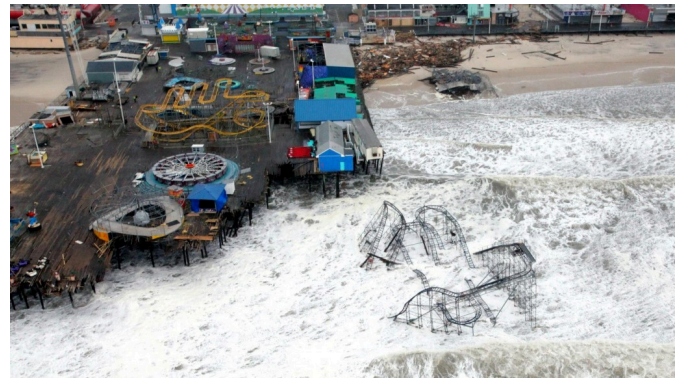
Figure 19.3.2 Damage to the Casino Pier, Seaside Heights, New Jersey, from Hurricane Sandy, November 2012.
