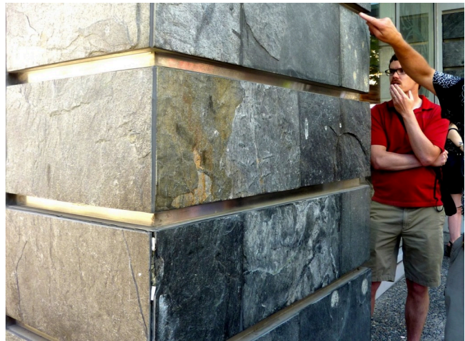
Figure 20.2.3 Slate used as a facing material on a concrete building column in Vancouver.
