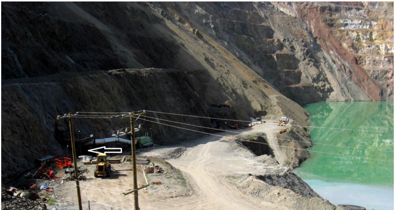
Figure 20.1.9 Entrance to an exploratory decline (white arrow) for the New Afton Mine situated in the side of the open pit of the old Afton Mine, near Kamloops, B.C.
