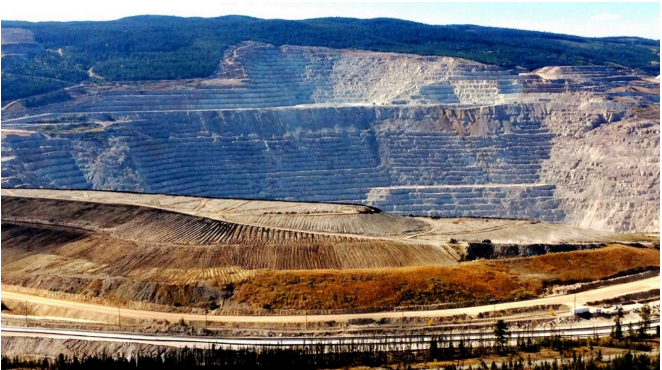
Figure 20.0.1 The open pit (background) and waste-rock piles (middle) of the Highland Valley Copper Mine at Logan Lake, British Columbia.
