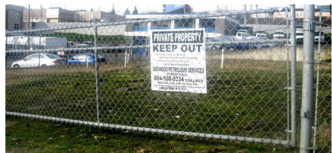
Figure 14.4.8 A closed and fenced gas station site in Nanaimo, B.C. The white pipes in the background are wells for monitoring groundwater contamination on the site.
