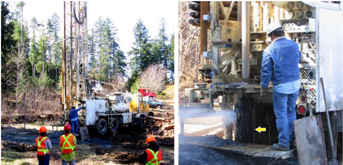
Figure 14.3.1 A water-well drilling rig in operation near Nanaimo, B.C. In the photo on the right the well is being test-pumped with air pressure. The casing (yellow arrow) is about 40 centimetres in diameter.
