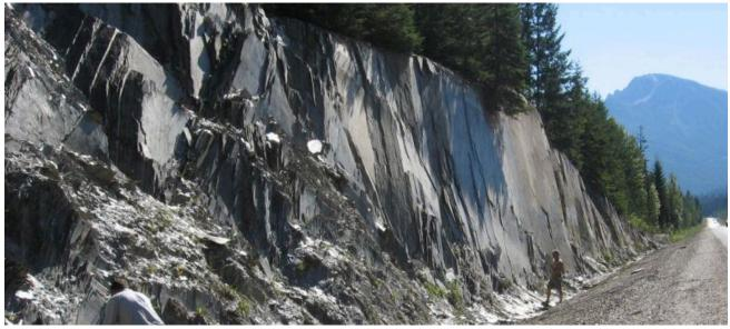
Figure 5.1.2 Exfoliation of slate at a road cut in the Columbia Mountains west of Golden, B.C.
