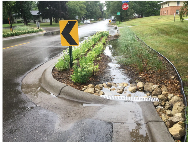
Figure 9.3 Example of a vegetated bioswale
