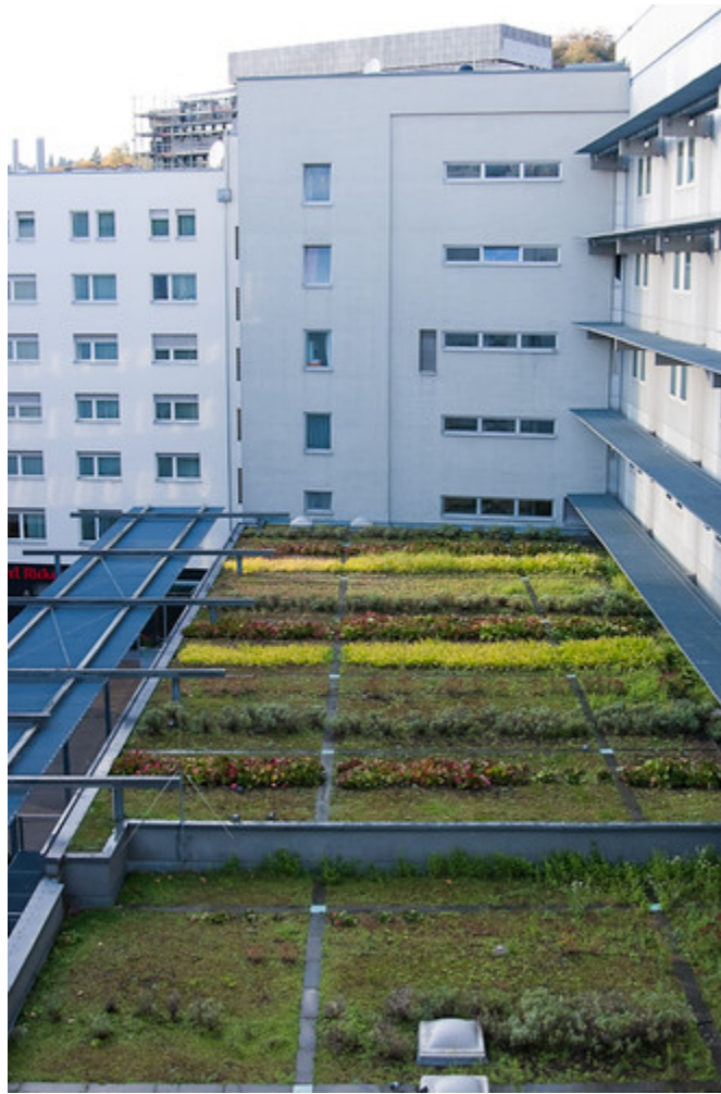
Figure 9.1 Example of an extensive green roof
