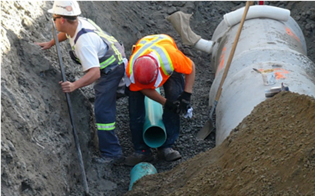
Figure 10 Installing two pipes in one trench
