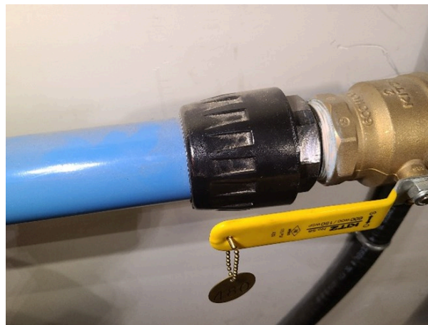
Figure 4b Aluminum compressed air fittings
