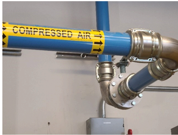
Figure 4a Aluminum compressed air fittings
