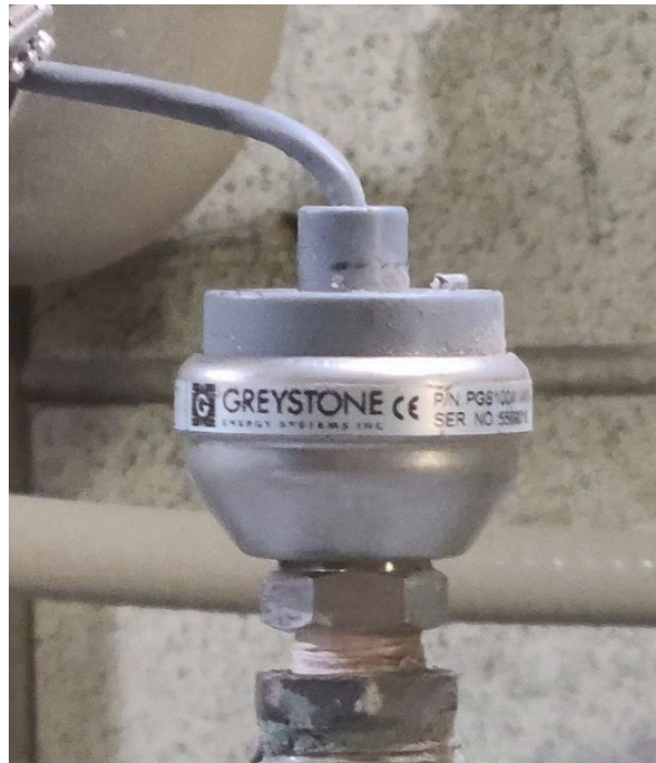
Figure 1a Pressure sensor
