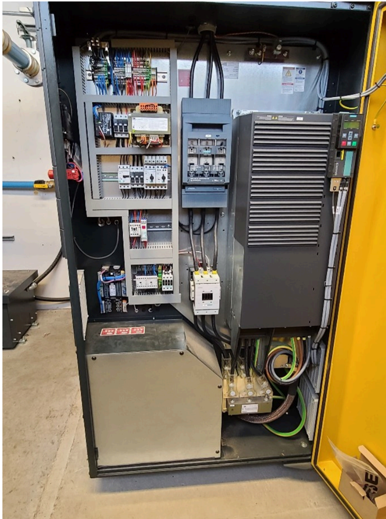
Figure 6 Compressor self contained electronic controls chamber
