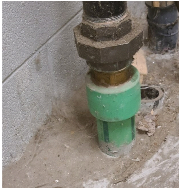
Figure 3 Polypropylene (PP) underground compressed air line
