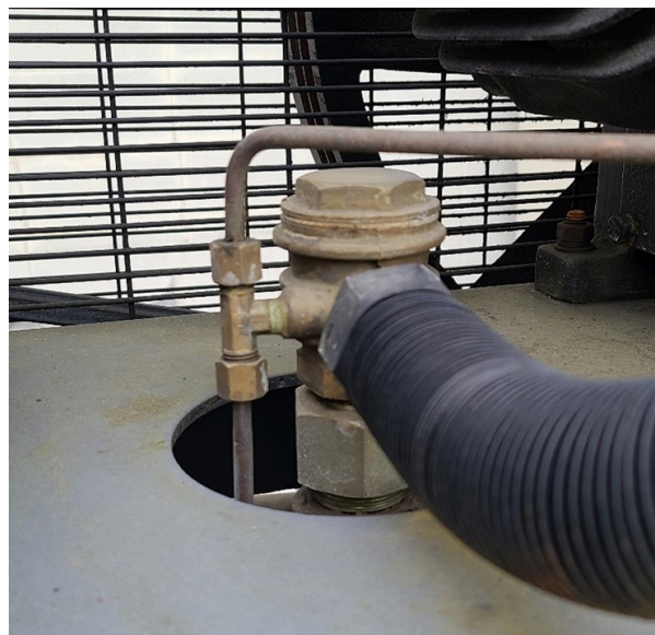
Figure 3 Angle check valve with pressure switch/unloading line connection
