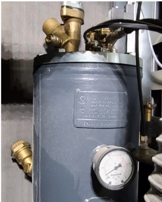
Figure 3 Oil separator (left) and cartridge components (right)
