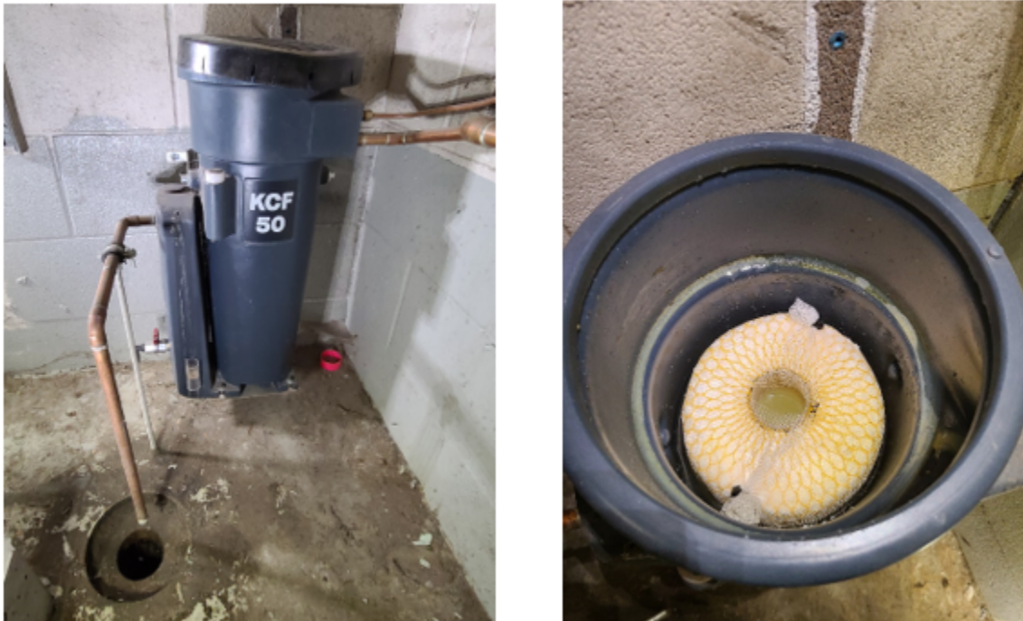
Figure 8 Oil/water separator
