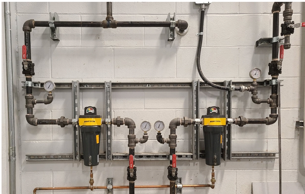
Figure 34 Secondary filter bank
