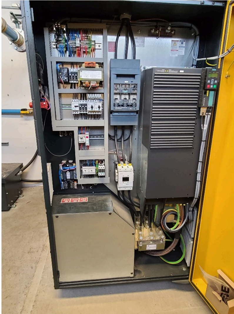
Figure 6 Compressor self contained electronic controls chamber
