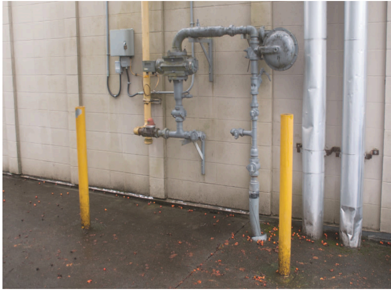
Figure 18 Pipe bollards filled with concrete protecting gas piping
