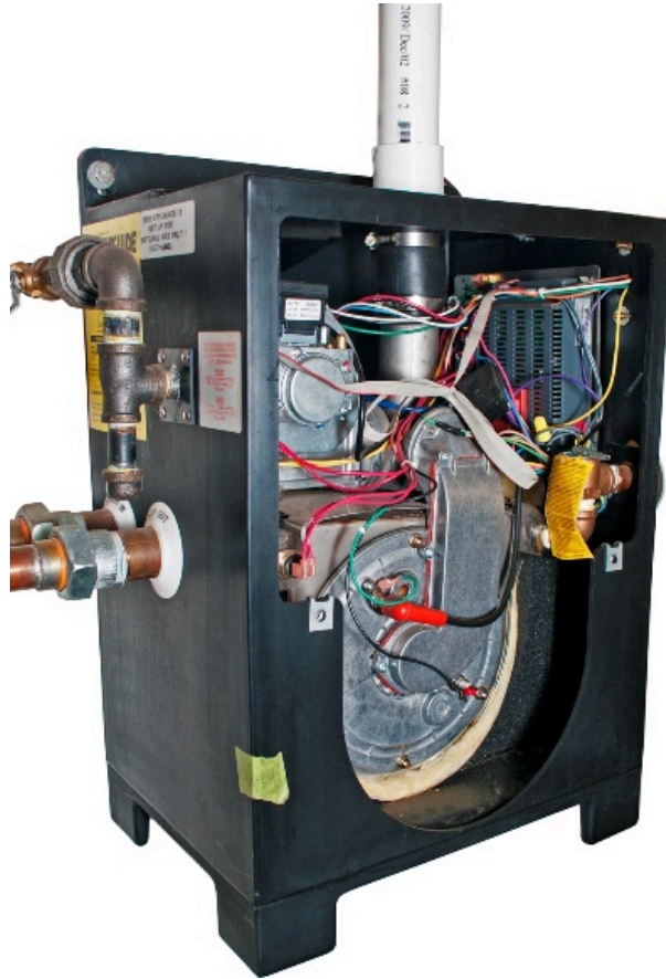
Figure 2 Small residential condensing boiler
