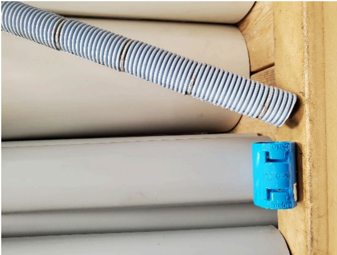
Figure 9 Flexible PVC conduit and coupling
