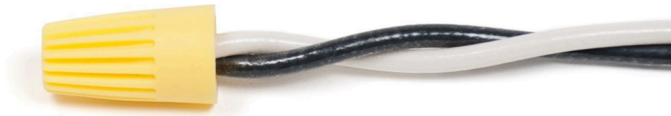
Figure 5 Twist-on connector installed
