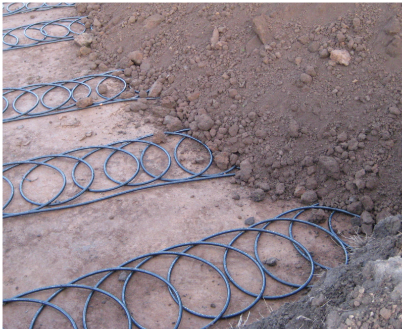
Figure 6 Partially backfilled “slinkies”
