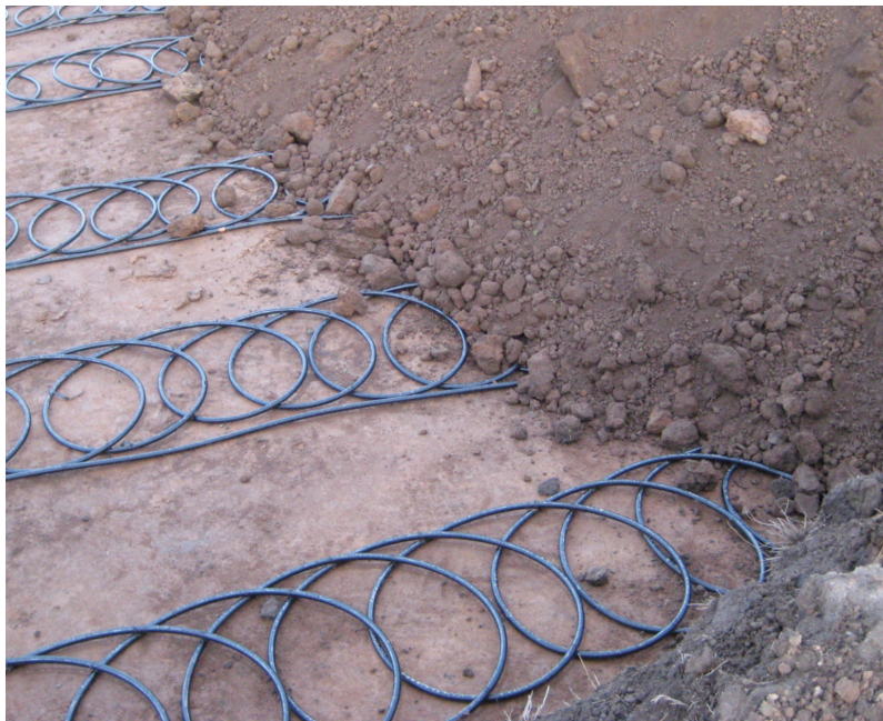
Figure 6 Partially backfilled "slinkies"
