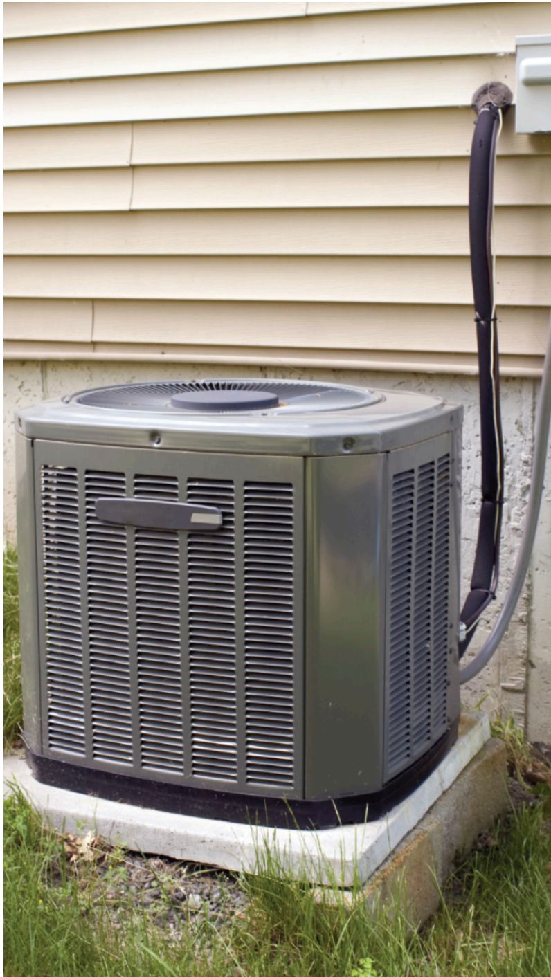
Figure 4 Typical air-to-air outdoor unit
