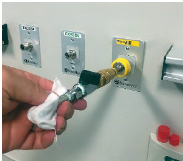
Figure 2. Piping purge being performed at a terminal unit
