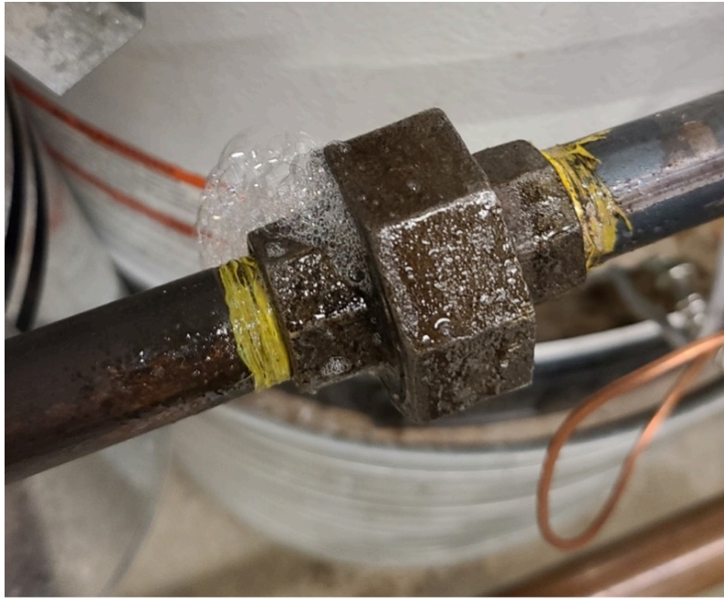
Figure 5. Leaking joint
