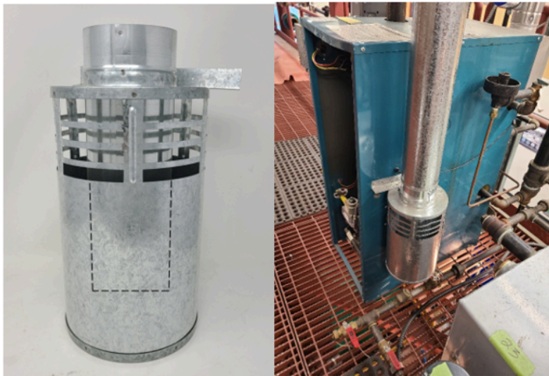
Figure 18. Combustion air pot/bucket
