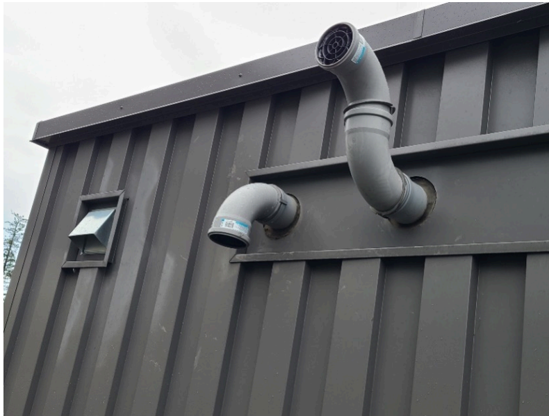
Figure 19. Direct vent terminations
