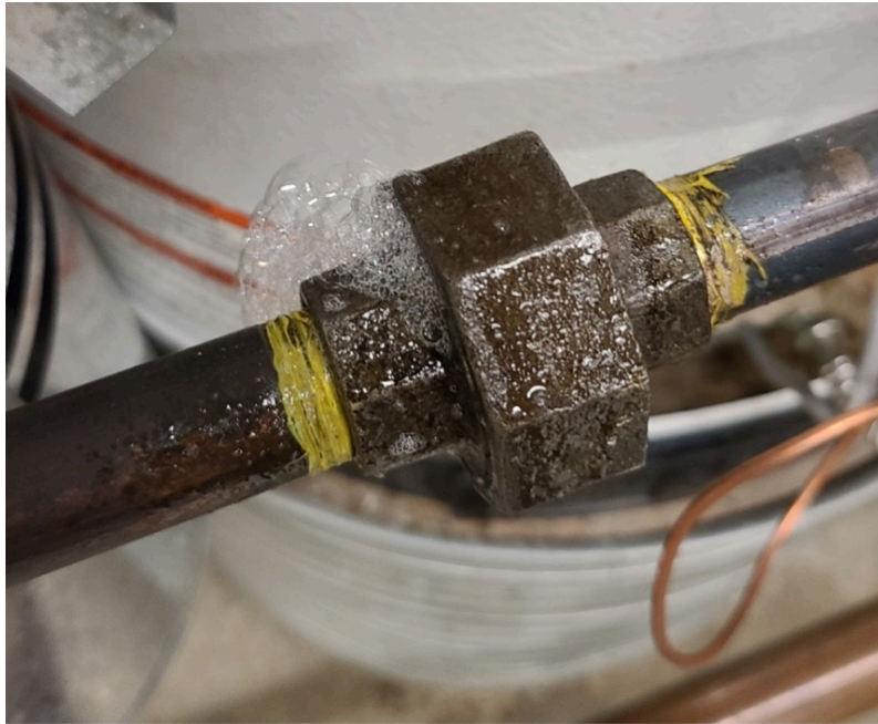
Figure 5. Leaking joint
