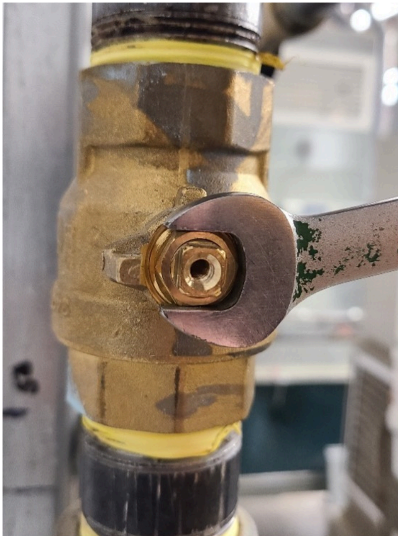
Figure 4. Tightening ball valve packing nut
