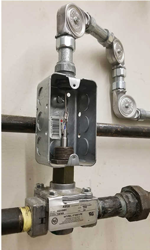
Figure 90. Kitchen exhaust fire extinguishing system
