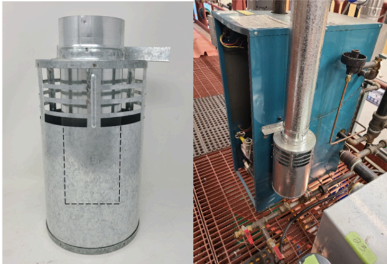
Figure 18. Combustion air pot/bucket
