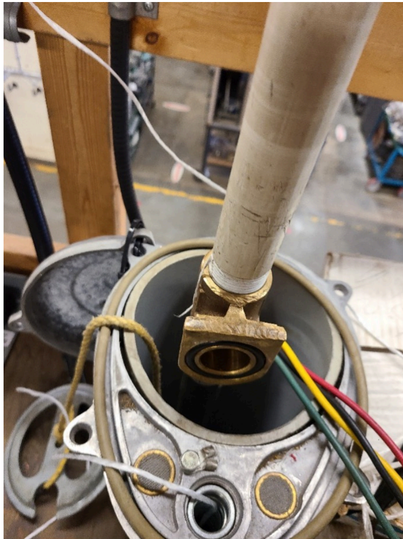
Figure 60. Well cap and pitless being installed
