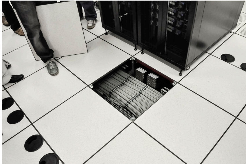
Figure 18. Cellular floor tile removed for access to wires and cables
