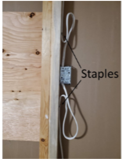
Figure 30. Staples and wire loops near box
