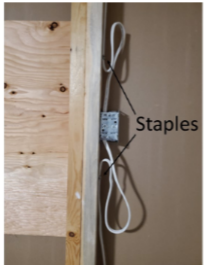
Figure 30. Staples and wire loops near box
