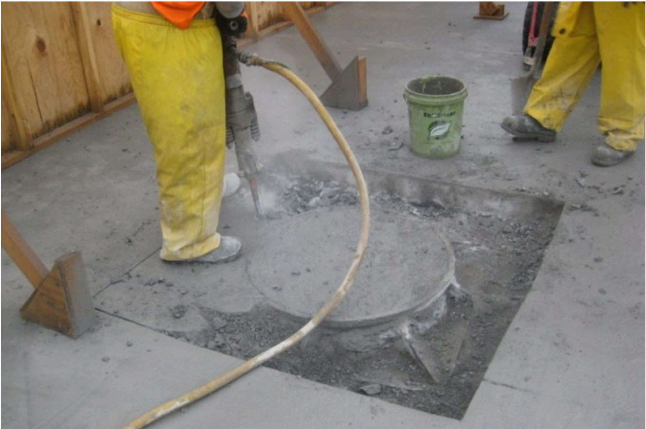
Figure 24. Repair of a manhole
