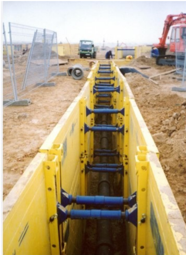
Figure 20. Trench box shoring
