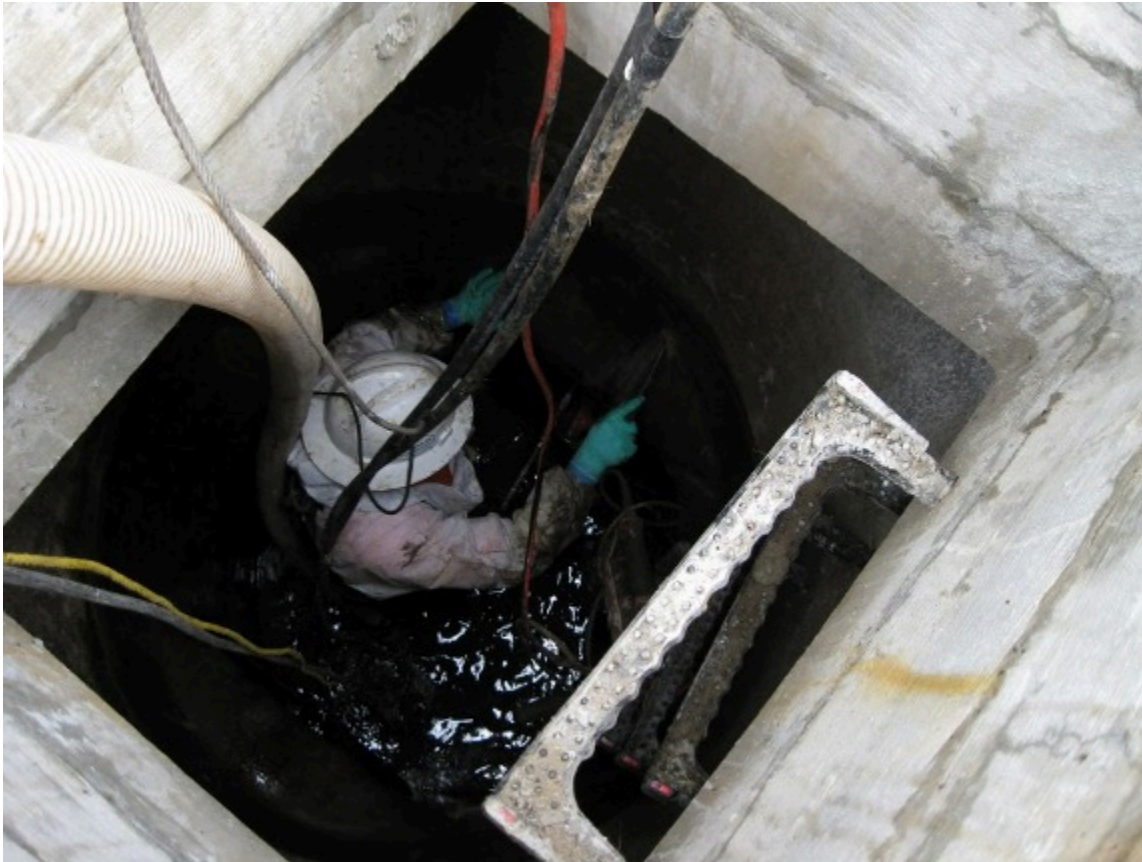
Figure 22. Authorized worker entering a catch basin
