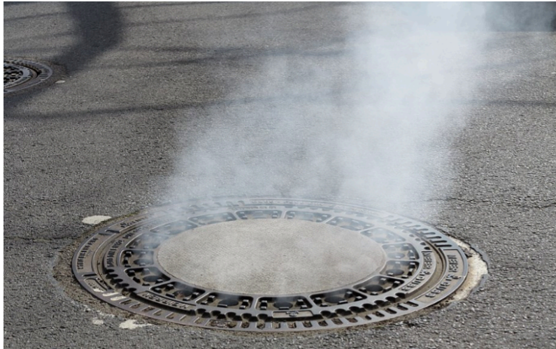
Figure 14. Smoke testing a sewer
