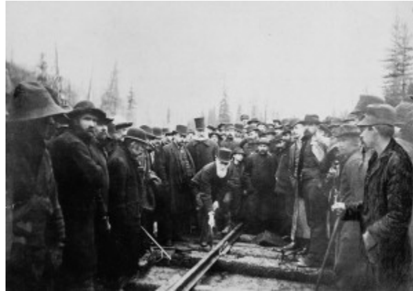
Figure 8.1 Driving home the last spike of the CPR, 7 November 1885.
