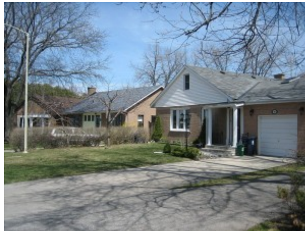
Figure 9.58 Suburbs have been criticized for “cookie-cutter” housing designs. In places like Don Mills, where the influence of the 1920s Garden City movement and modernist architecture can be seen, the whole design was in fact tightly controlled as a kind of social experiment in creating a livable space.
