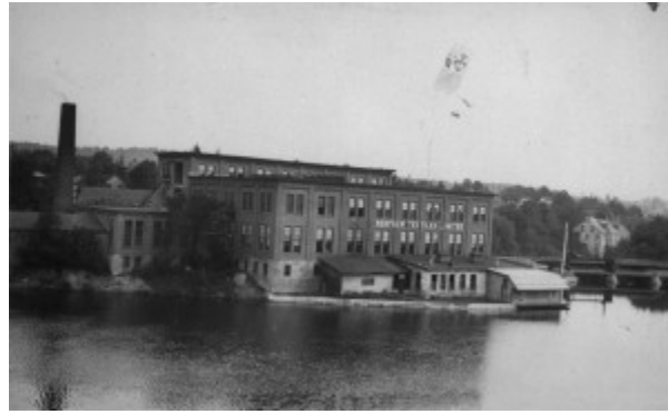
Figure 3.23 The clean lines of brick factories, the bold smokestacks and water towers, and the promotional branding visible on this textile mill were all indicators of industrial progress and capitalist confidence in central Canadian communities like Renfrew, Ontario.
