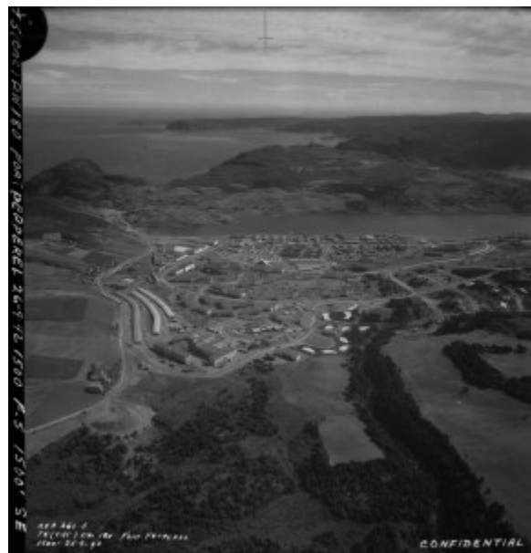
Figure 9.6 Building the massive American Fort Pepperell provided jobs to hundreds of Newfoundlanders and confirmed a United States presence in the former Dominion that drew it into the orbit of Washington.
