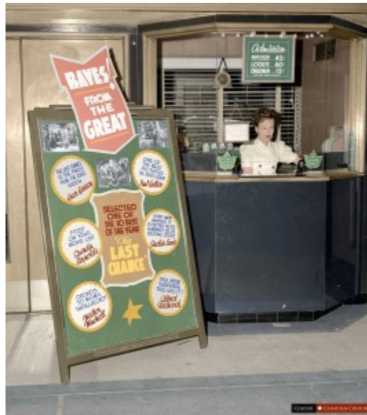
Figure 10.29 In 1945, the city centre cinemas were still thriving. Shows were usually continuous, hence the saying, “this is where I came in.”
