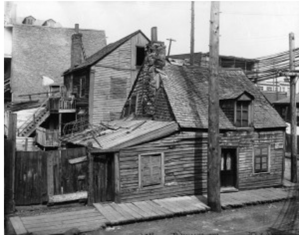
Figure 3.27 A survey of working-class housing in Montreal in 1903 found high density and badly deteriorated conditions.
