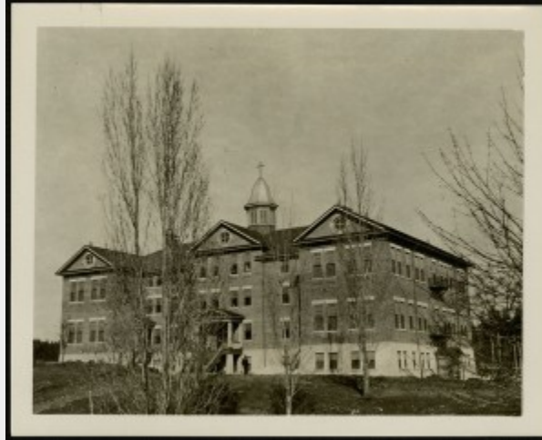
Figure 11.19 Kuper Island Residential School.
