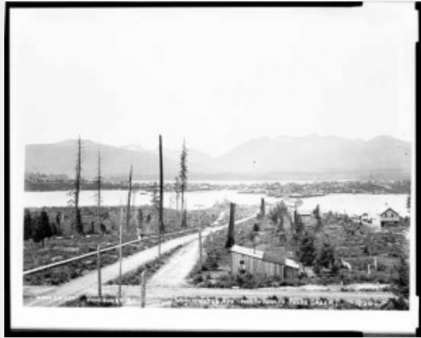
Figure 8.25 The False Creek mudflats at high tide in 1890, only recently denuded of trees but still a salmon spawning ground and a source of clams.
